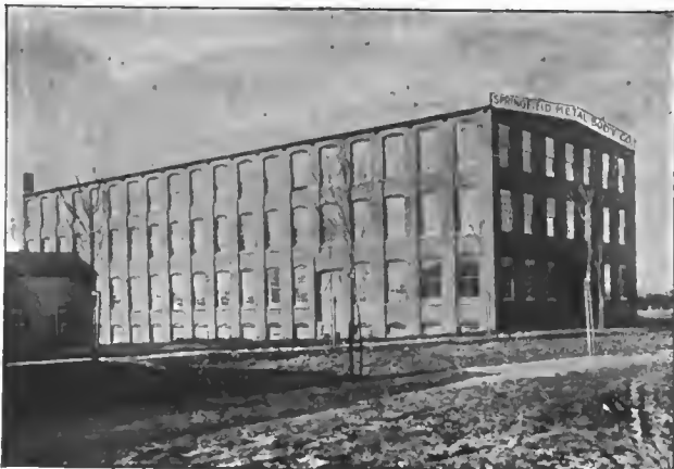
NEW ADDITION TO SPRINGFIELD METAL BODY CO.'S PLANT.
